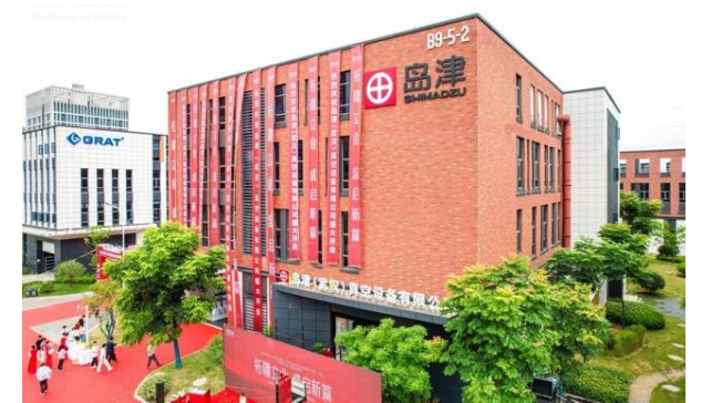
Service base in Wuhan, China, established in June 2023
