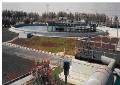
Fig. 5. Clarifier at Rahima STP
