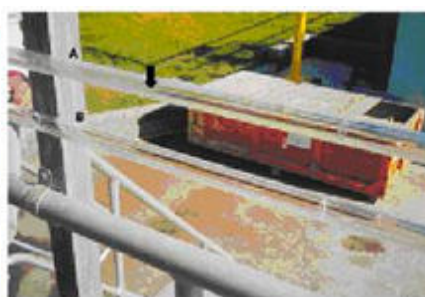
Fig. 12. UV lamp quartz tubes; A is tube partially cleaned; B is cleaned tube
